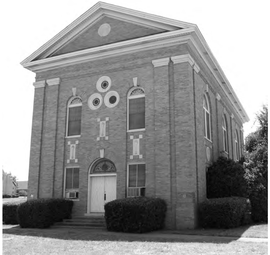
Arlington Heights Masonic Lodge 1184 was built in 1922 making it one of the oldest buildings on Camp Bowie Boulevard.
