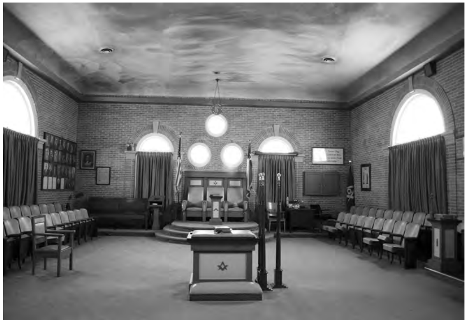
The Lodge Hall on the second floor is a breathtaking expanse of a room, dominated by a curved lathe-and-plaster ceiling, painted sky blue with white clouds and studded with brass stars. Most of the original wooden bench seats were handed down to other lodges years ago, but several original quarter-sawn white oak chairs remain.
