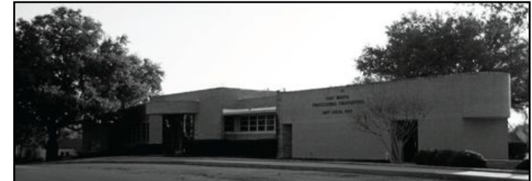
In late 2009, the Fort Worth Professional Firefighters Association completed their move into the former Medical Arts Building at 3855 Tulsa Way.
